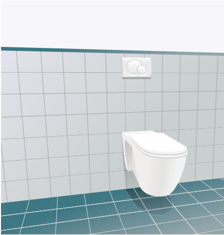
Mount the flush plate and wall-hung toilet.
